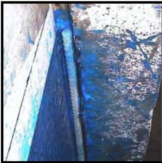
**(c) Inserting a glass FRP bar**
