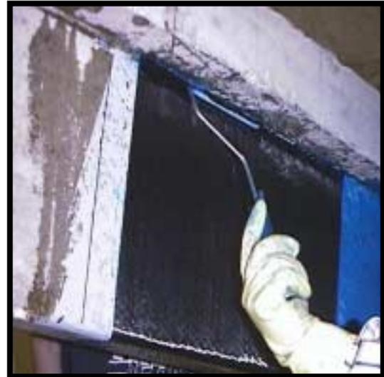
**(b) Applying CFRP sheet**
