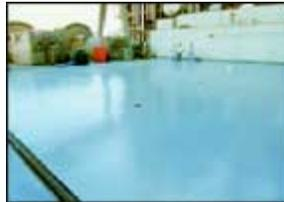
The turbine deck of Ocean Vista Power Generation Station in Oxnard, California consists of a post-tensioned concrete deck, supported by structural steel framing, that was built in 1957 in conjunction with the turbine generator pedestal. Concerns over the safety of the deck had come from noticeable cracking and spalling of the concrete and visible corrosion of the post-tensioning cables.
